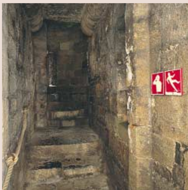
Above and opposite: The introductory sign and examples of warning signs in position at Caernarfon Castle.
