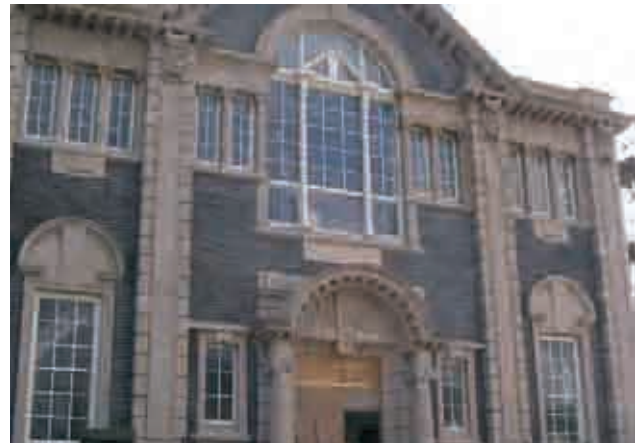
Tabor Chapel, Maesteg, Glamorgan, before (left) and after (above) restoration with grant aid as part of a Townscape Heritage Initiative Scheme.
