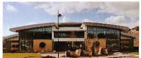
One of the new quality, energy efficient buildings at Tredegar Business Park – Phase I.
